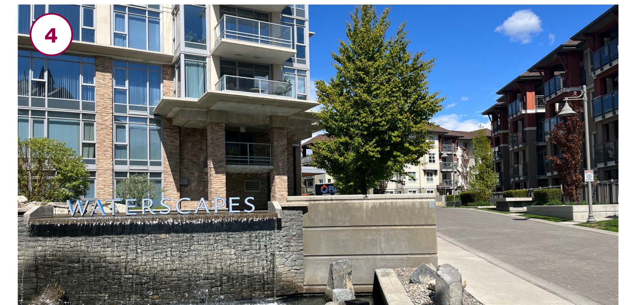
4 West entrance onto Private Street at the completed Waterscapes Phase 1, from Sunset Drive.
